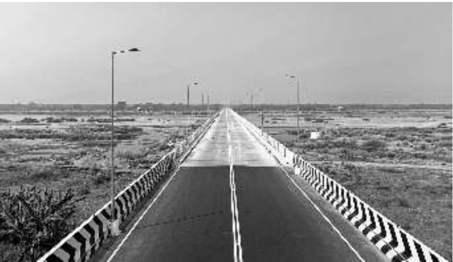
Vital link: The new bridge built across the Cauvery between Nerur in Karur district and Unniyur in Tiruchi district. SPECIAL ARRANGEMENT
