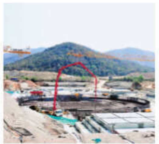
The quarry site for Kaiga Units 5 and 6
