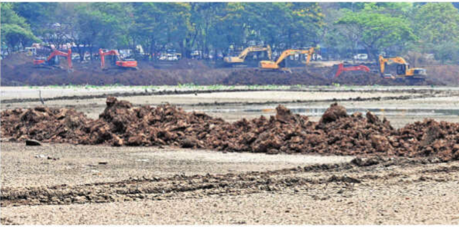
Ahead of the monsoon, desilting work on in full swing at the dried up Hebbal Lake on Monday | SHASHIDHAR BYRAPPA
