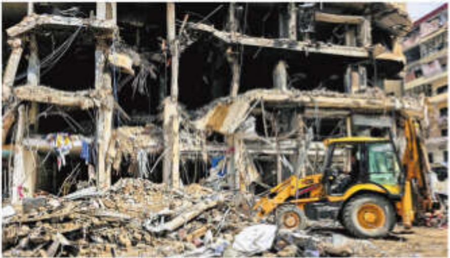
A bulldozer clears rubble from a street at the site of an Israeli airstrike in Beirut's southern suburbs | AFP
