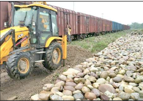
In this handout photo released by the NFR, workers reinforce railway tracks as part of strategic preparedness measures for the monsoon season. (Photo Courtesy: CPRO NFR)
