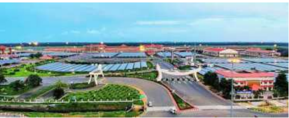
The airport currently operates cargo warehousing facilities spread across approximately 2.5 lakh square feet. FILE PHOTO
