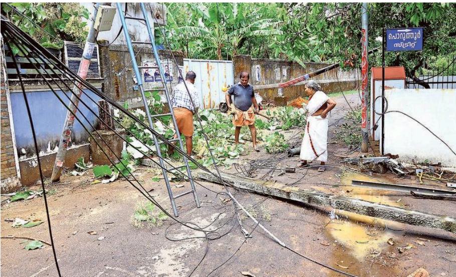
Heavy damage: Electric poles and trees lie uprooted following downpour and strong winds at Vidya Nagar Street in Ancheri, near Thrissur, on Wednesday night. K.K. NAJEEB
