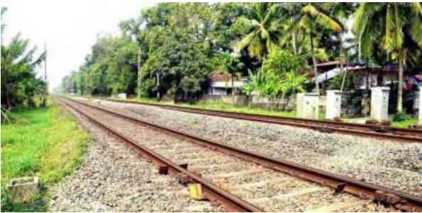
Cause for concern: The repeated fatal accidents have prompted both the Railway Protection Force and the Government Railway Police to enhance safety measures and awareness drives along vulnerable stretches. FILE PHOTO
