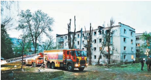
A residential building is seen damaged after a Russian strike on Dnipro, Ukraine.
