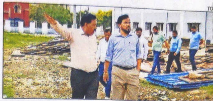
Patna Municipal Corporation commissioner Yashpal Meena inspects the ongoing work of Mandiri Nala on Tuesday
