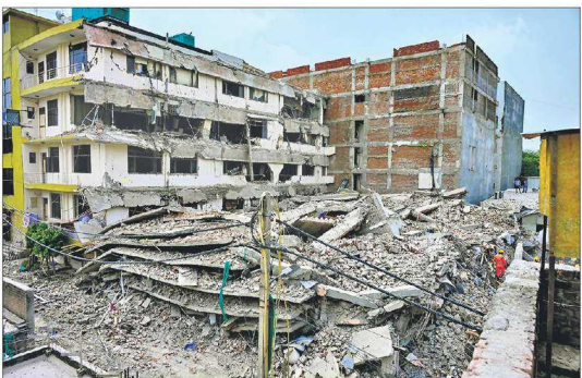
The death toll in the collapse of a commercial building near Saket Metro station in south Delhi rose to six on Sunday, while several others were rescued from the debris and admitted to hospitals, officials said. Delhi Police has registered a case under relevant sections, including culpable homicide. The Municipal Corporation of Delhi has suspended two engineers over alleged lapses.
