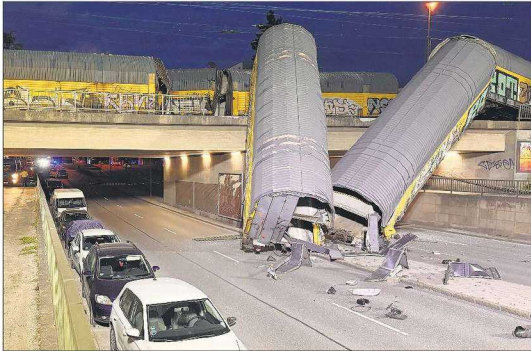
Two cars of a freight train derailed after a collision and fell off a bridge in Munich, Germany, June 20. One person was killed. The cause of the incident is under investigation.
