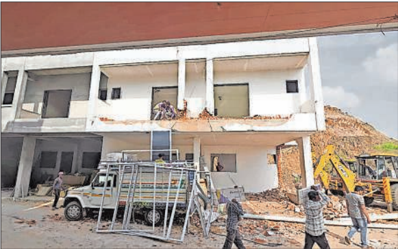
The demolitions being carried out at Garudeshwar, in Narmada district, Gujarat, on Sunday. EXPRESS
