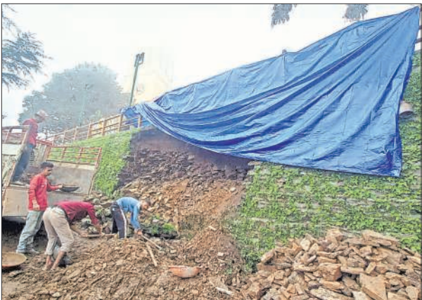
Breast wall restoration work underway near Christ Church at the Ridge in Shimla on Tuesday. EXPRESS
