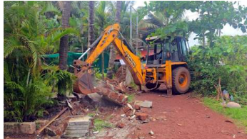
A bulldozer begins demolishing structures in Temwada-Morjim. Nivrutti Shirodkar
