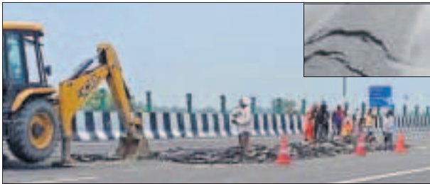
Repair work undertaken after a road surface damage was reported near Korari in Unnao, barely 3 weeks after the expressway was opened to traffic. (Inset) The damaged portion.
