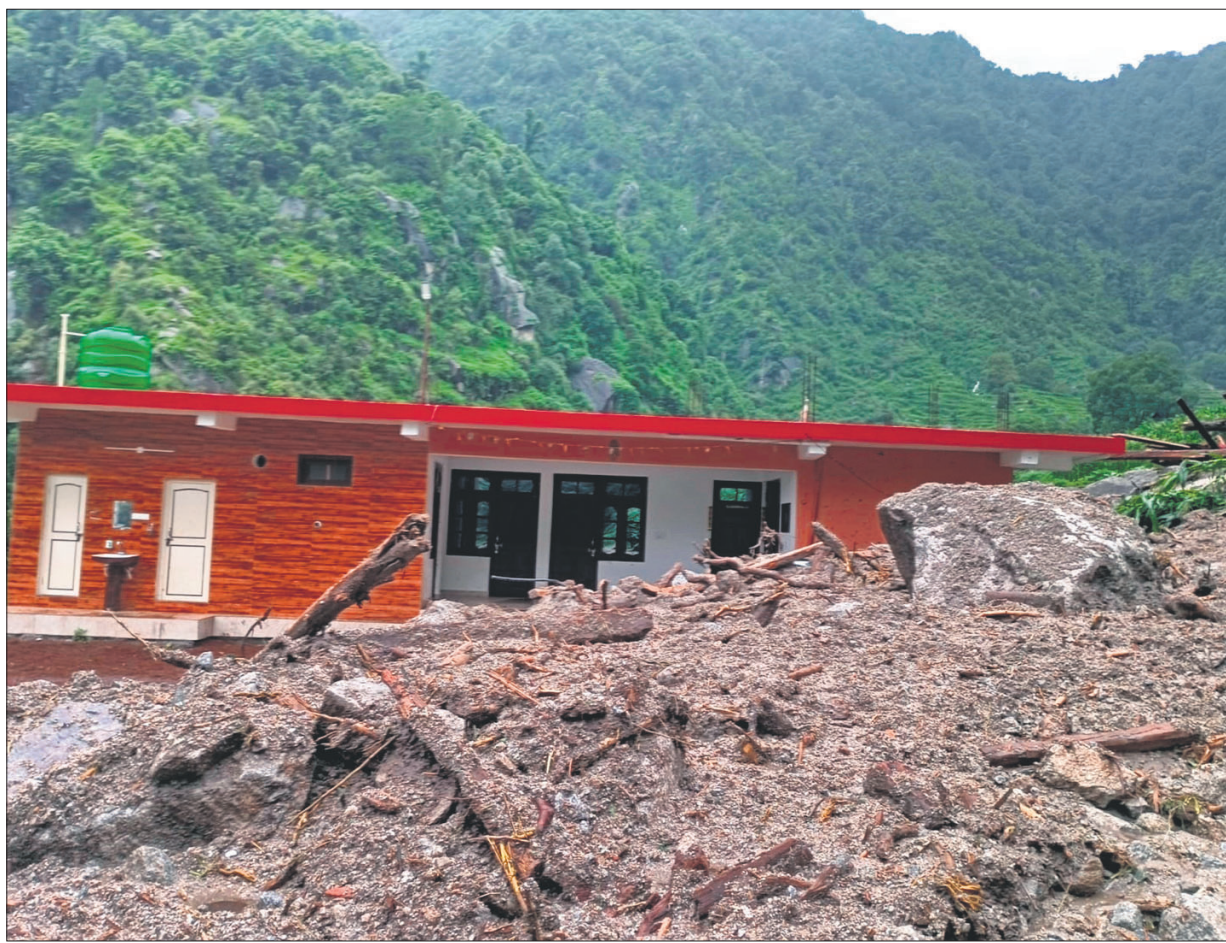
Devastation caused due to a landslide triggered by heavy rain in the Boh area of Shahpur in Kangra district.
