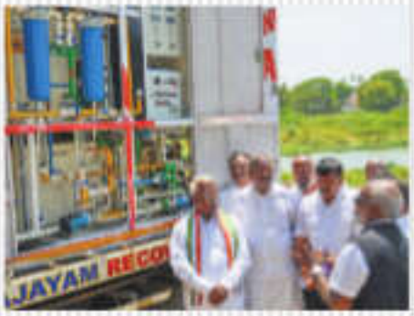
C Robert Bruce, MP, and others during the demo of the sewage treatment system | V KARTHIKALAGU
