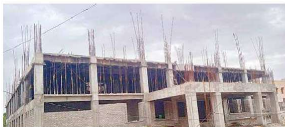
The critical care unit being constructed at the Area Hospital in Rayachoti
