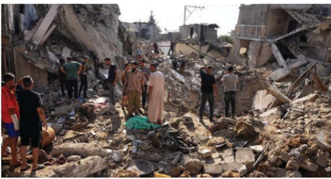
Palestinians inspecting destroyed buildings at the scene of an Israeli airstrike, at al-Maghazi refugee camp, central Gaza Strip
