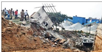
According to preliminary information, plant owner and other employees were not present when the accident occurred
