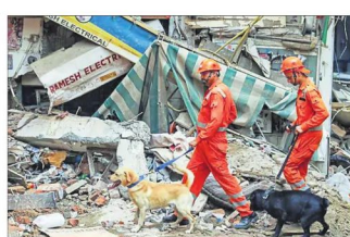
Rescue and search operations underway after a five-story building collapsed at Satya Niketan near South Campus in New Delhi on Monday.
