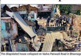
The dilapidated house collapsed on Vadva Panwadi Road in Bhavnagar
