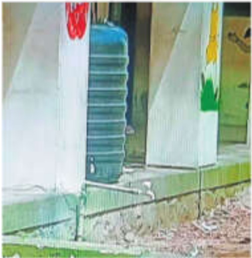
The water tank at the government primary school in Dindigul, in which excreta was found | EXPRESS
